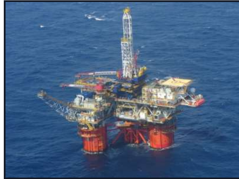
ATP Titan is the world's first multi-column deep draft reusable floating drilling and production platform
