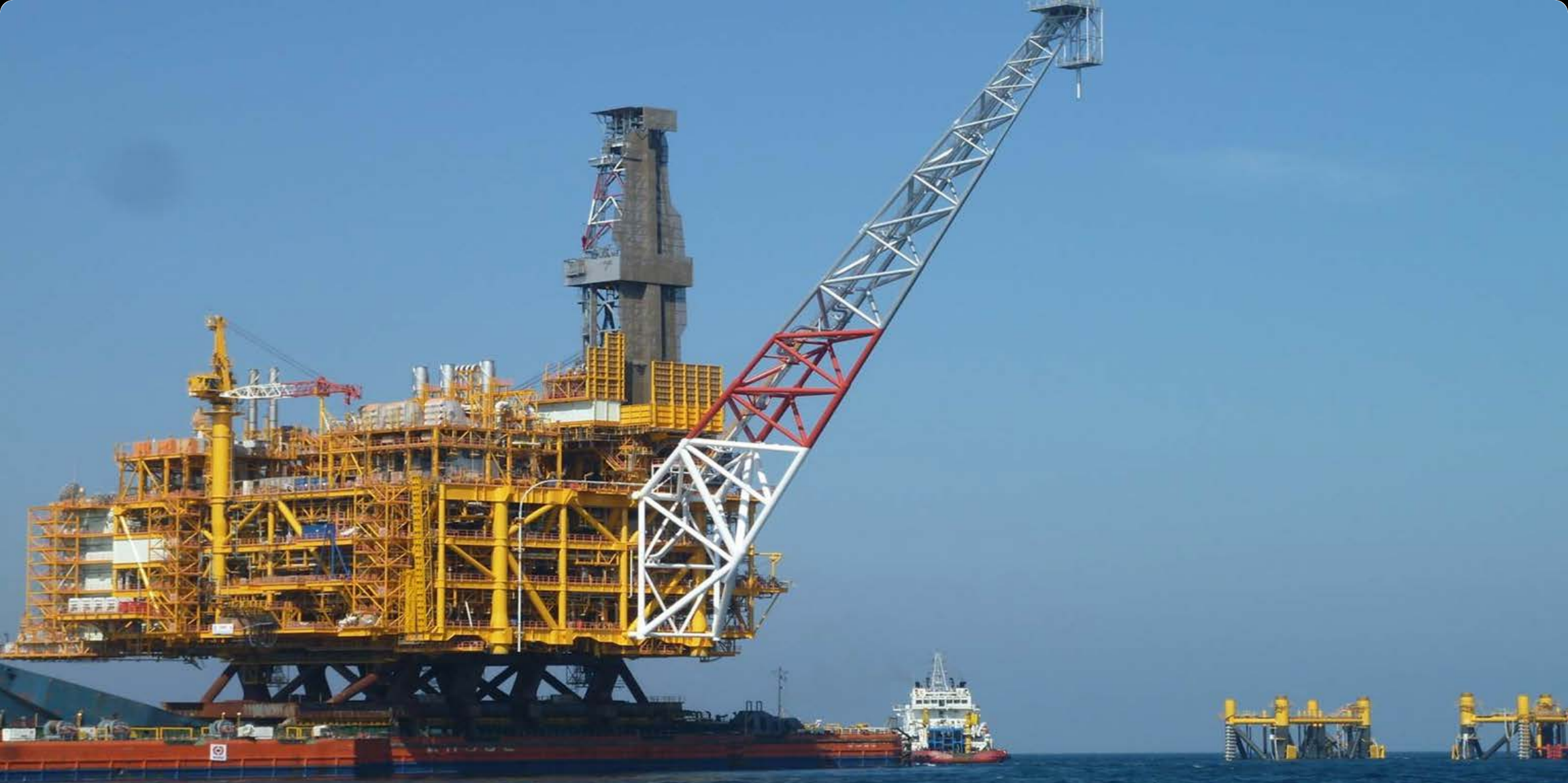
DAEWOO OIL/HYUNDAI HEAVY INDUSTRIES SHWE 26,000 mT topside float-over installation (2012)
