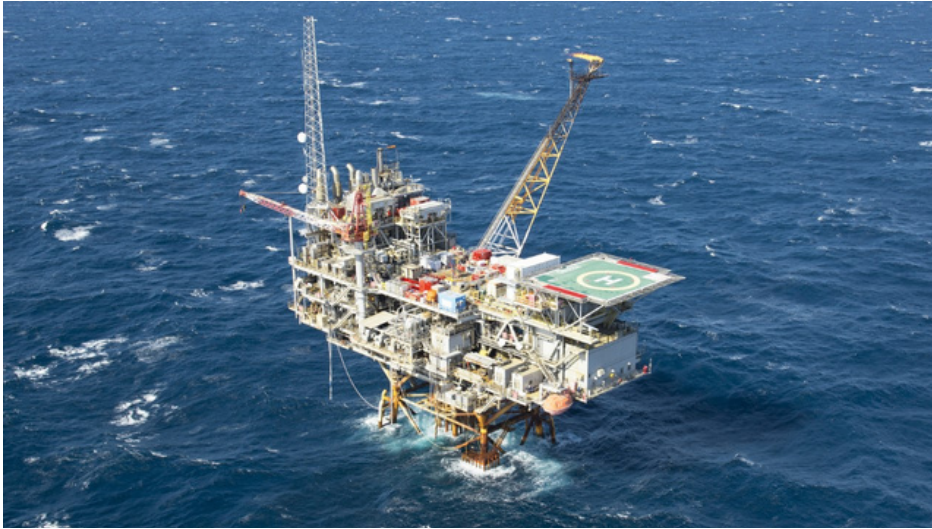
Shell's Enchilada platform
